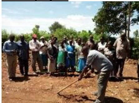
Breaking the ground of the St Patricks Prim School kitchen.
